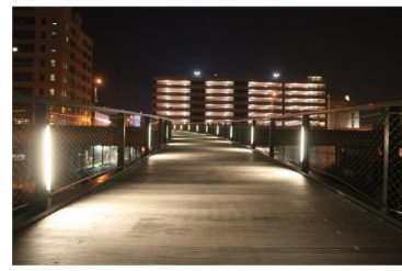
EXPOSED VERTICAL LIGHTS
