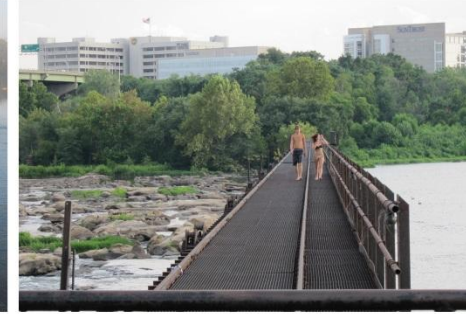
INFORMAL USE OF BROWN'S ISLAND DAM
