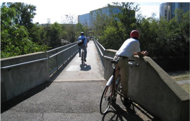
SUN TRUST PEDESTRIAN BRIDGE
