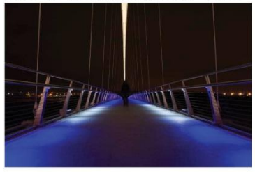
EXPOSED DISCREET PATHWAY LIGHTS
