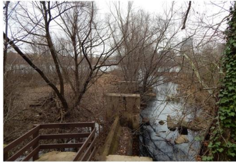
EXISTING PIERS, FROM MANCHESTER EMBANKMENT
