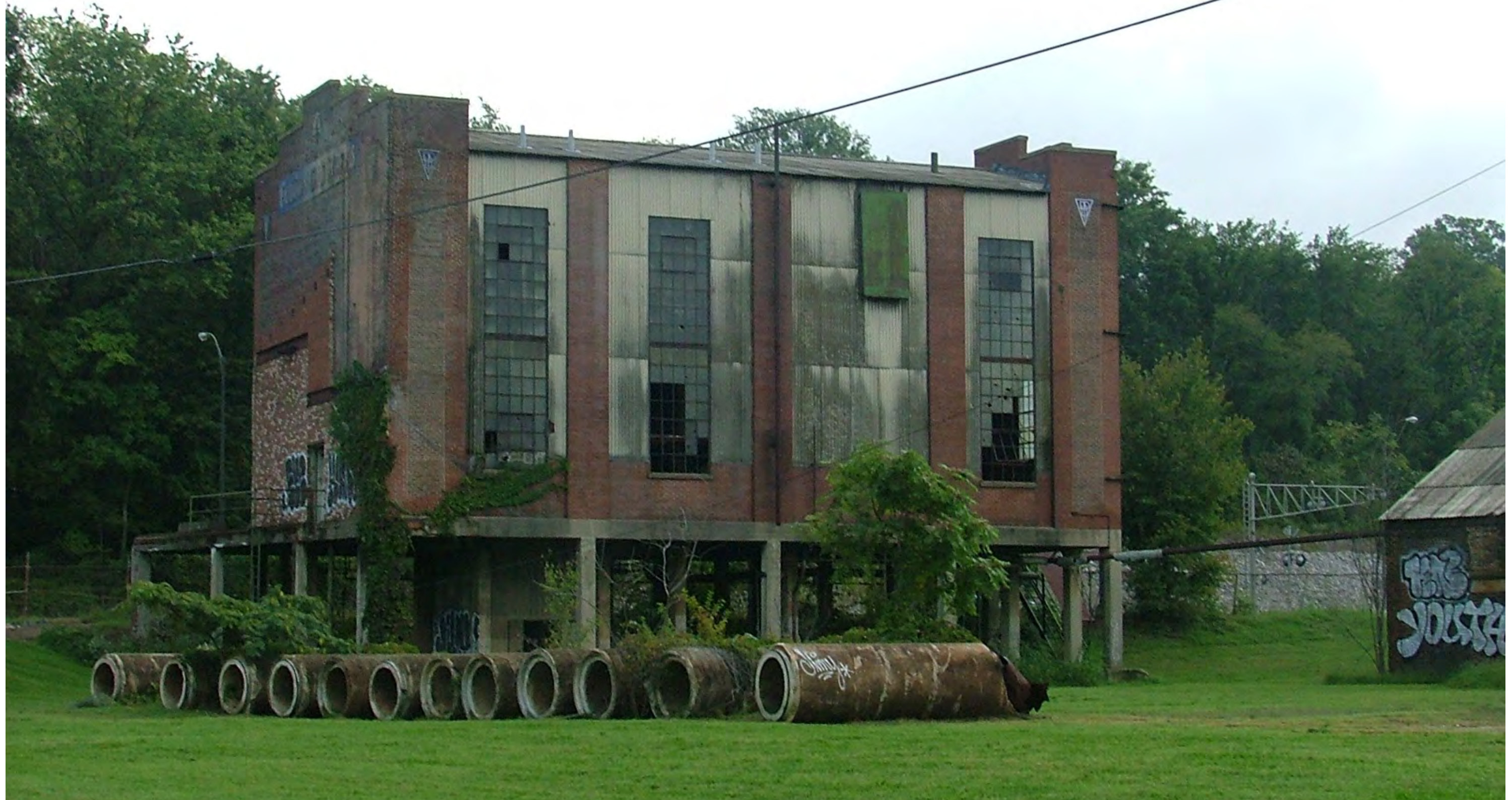
FULTON GAS WORKS: EXISTING CONDITIONS
