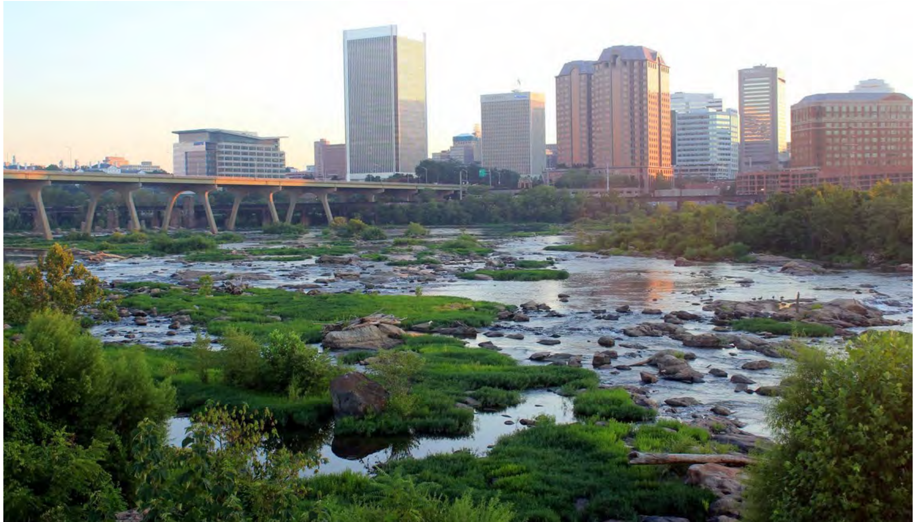
MANCHESTER: VIEW FROM FLOODWALL WALK, LOOKING NORTH TOWARDS DOWNTOWN RICHMOND
